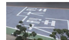
Heat insulating pavement (reducing road surface temperature by reflecting infrared rays)
