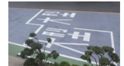
Heat insulating pavement (reducing road surface temperature by reflecting infrared rays)
