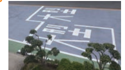
Heat insulating pavement (reducing road surface temperature by reflecting infrared rays)
