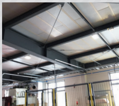
Thermal insulation of worksites with Thermax
