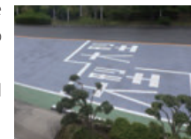
Heat insulating pavement (reducing road surface temperature by reflecting infrared rays)
