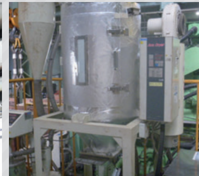
Toyohashi Plant / Heat insulation sheets as a measure for materials dryers
