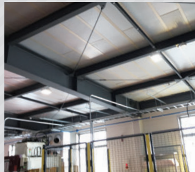
Thermal insulation of worksites with Thermax
