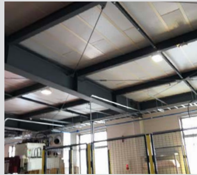
Thermal insulation of worksites with THERMAX
