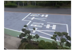
Heat insulating pavement (reducing road surface temperature by reflecting infrared rays)
