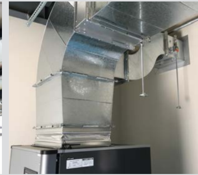
Utilizing heat exhaust from compressors
