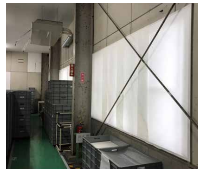
Applying CELL SHADE to windows
