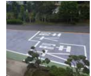
Heat insulating pavement (reducing road surface temperature by reflecting infrared rays)
