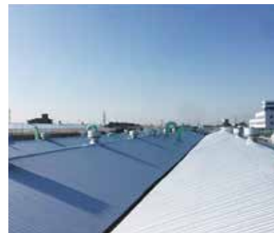
Anjo Plant: Heat insulation cover on plant roofs
