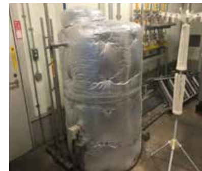
Affiliated companies: Installation of insulation jacket on tanks
