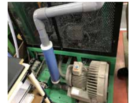
Kita-Kyushu Plant: Taking-out and taking-in of waste heat from fans
